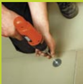
3. In addition, fix with 8 wood screws and 30mm washers per board the Multiboard on the wooden floor.
