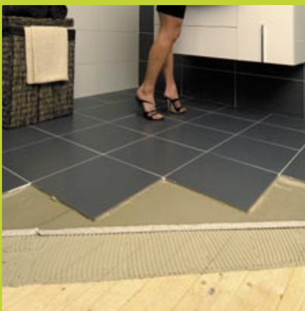
Multiboard as substrate for tile floors in order to reduce contact noise and to level the floor.
