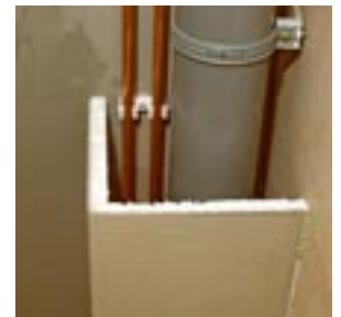
Very simple covering of pipes and drains.
