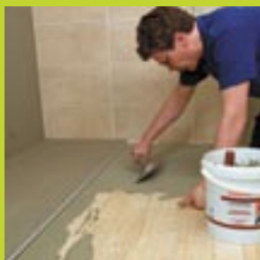
1. Apply on the flat floor Foby PF-Mortar.
