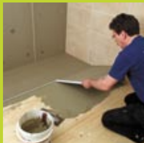
2. Lay the Multiboard in the PF-Mortar with staggered joints and let the PF-Mortar cure completely.
