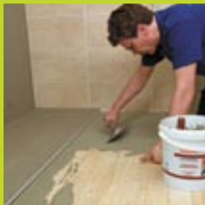
1. Apply on the flat floor Foby PF-Mortar.
