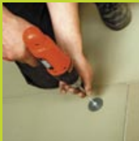
3. In addition, fix with 8 wood screws and 30mm washers per board the Multiboard on the wooden floor.
