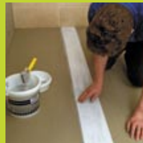
4. Apply self adhesive reinforcement tape on the joints and the washers.
